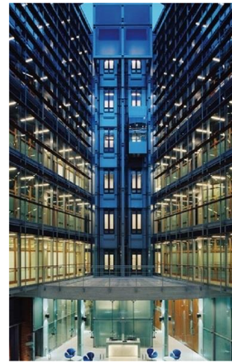
Projects @ Hopkins Architects GEK Group Headquarters
